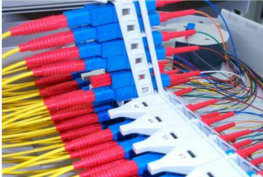
Figure 79. Installed New Adapter
