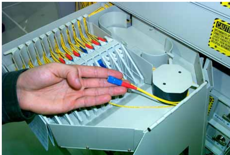
Figure 49. Patch Cord Routed To Rear Side of Adapter Pack
