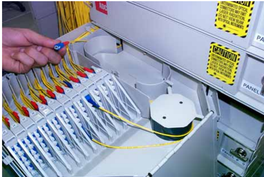
Figure 48. Patch Cord Routed To Left Rear Side of Open Drawer
