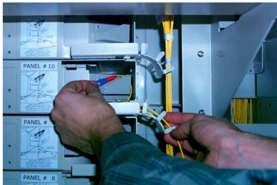
Figure 46. Connector Oriented Correctly for Placement in Fiber Transport
