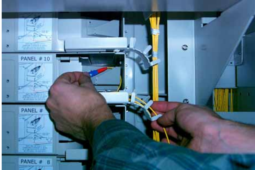
Figure 56. Connector Oriented Correctly for Placement in Fiber Transport
