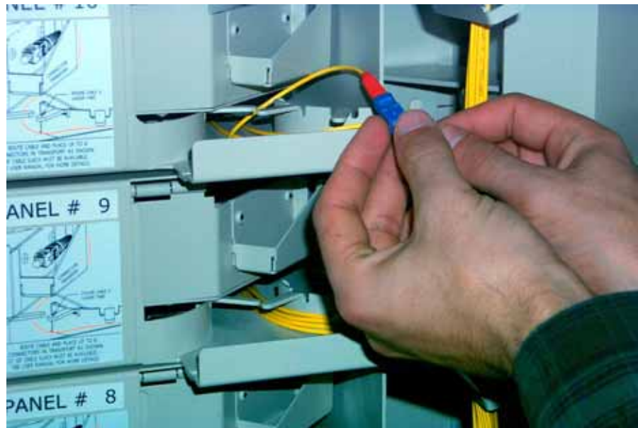
Figure 45. Positioning Patch Cord in Radius Limiters
