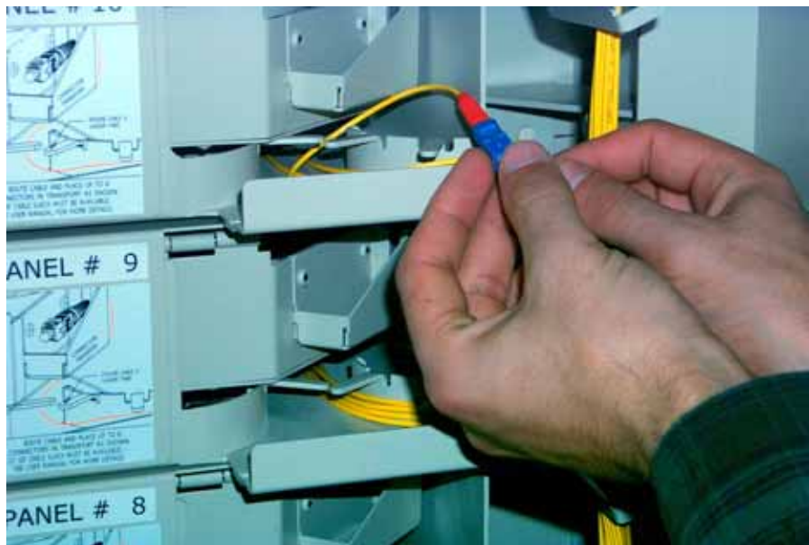
Figure 55. Positioning Patch Cord in Radius limiters
