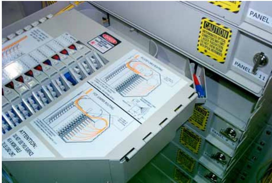
Figure 47. Connector in Fiber Transport When Hinged Drawer is Opened
