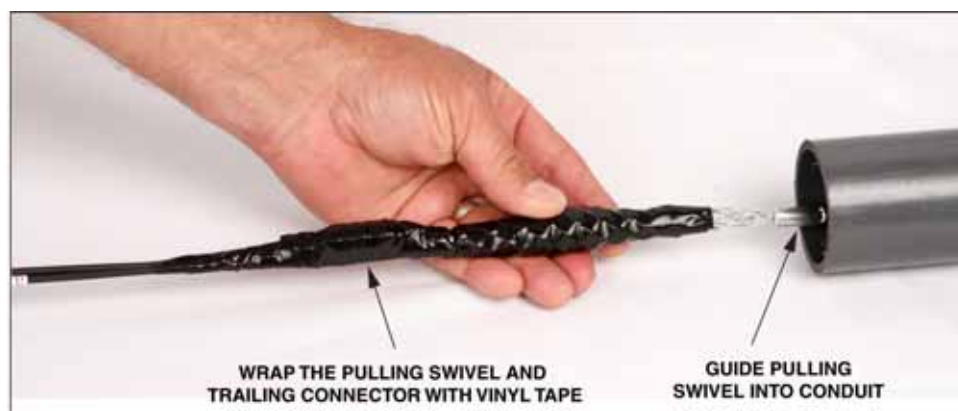
Figure 49. Wrap Pulling Swivel and Connectors with Vinyl Tape
